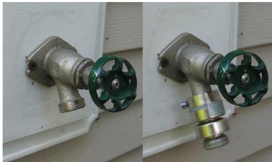
Hose bib with BFP; water supply is protected from contamination when a hose is connected.
